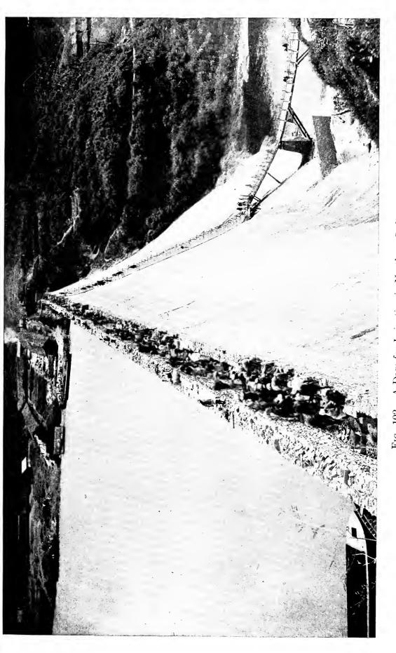
Note the great height of the dam. The flare at the bottom is the counterpart of a similar flare on the other side, and is needed to resist the vast weight of the water. Fig. 102.—A Dam for Irrigation in Northern India.
